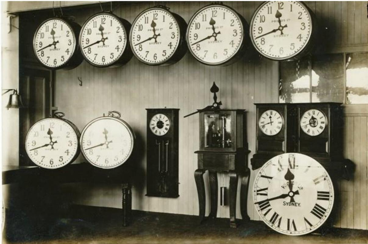
Some of the special electric self-contained clocks made to the order of the Sydney Harbor Trust, and installed on the various Ferry Jetties, Circular Quay.
